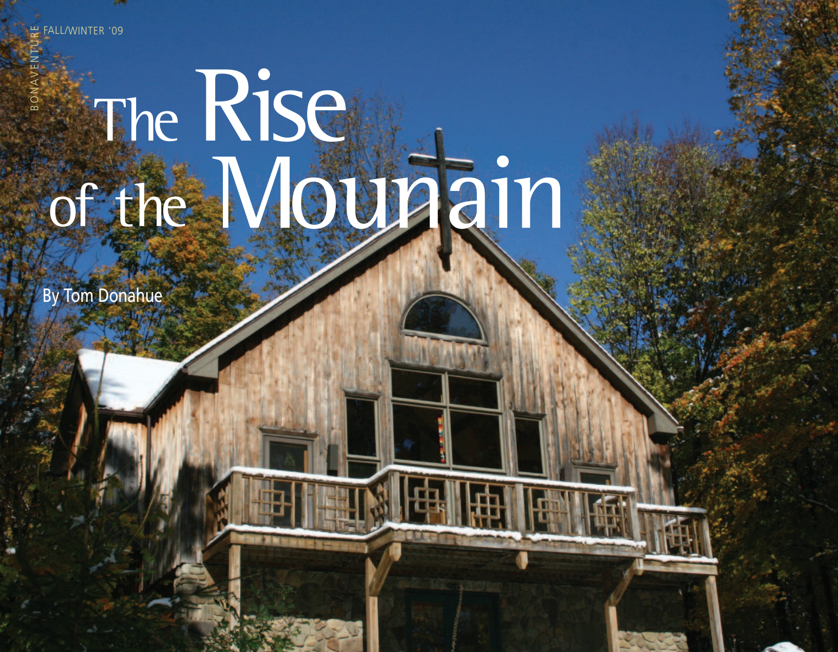
Holy Peace Chapel today (above) and under construction in 1988 (below, left)
