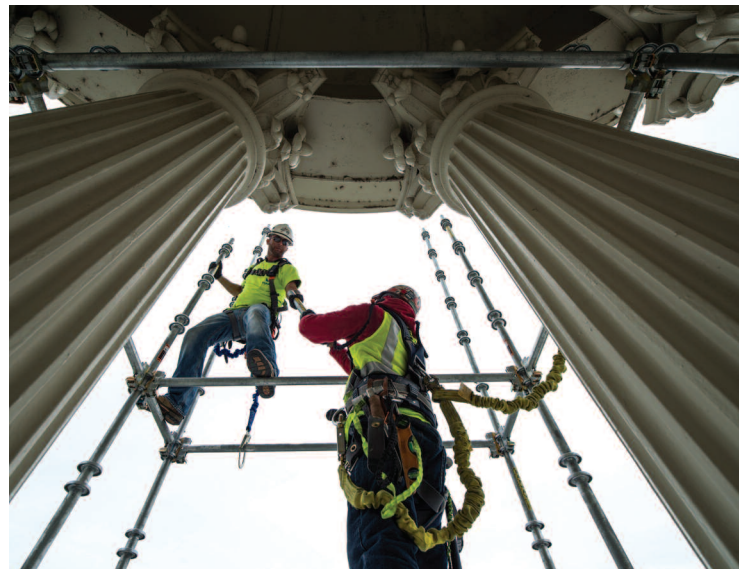
Workers climbed scaffolding hung from 52 miles of metal piping to remove paint and repair damage to the Capitol's dome.
